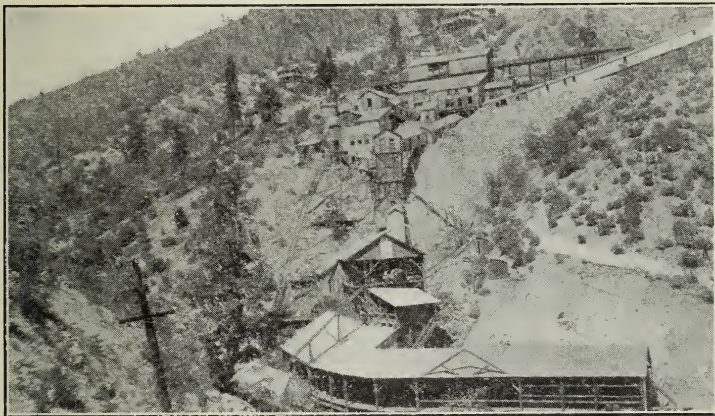
Crushing and Sizing Plant, Hornet Mine, Mountain Copper Company, Keswick, Shasta County.
