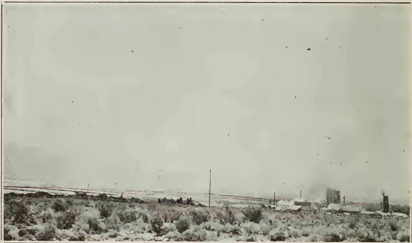
Inyo Chemical Company's Plant (formerly California Alkali Company), at Cartago, Owens Lake, Inyo County.
