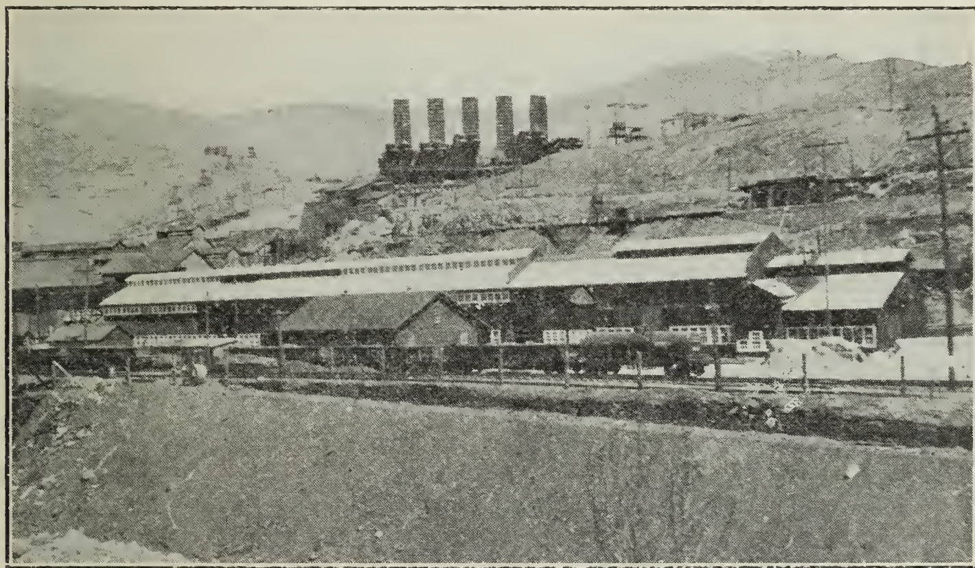
General View of Mammoth Smelter, Mammoth Copper Company, Kennett, Shasta County.
