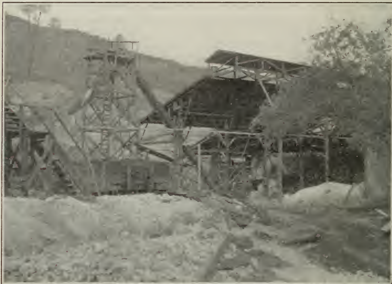
Calcining plant at the Sampson Magnesite Mine, west of Idria, San Benito County, California. Producing dead-burned magnesite in a rotary kiln. Photo by Walter W. Bradley.
